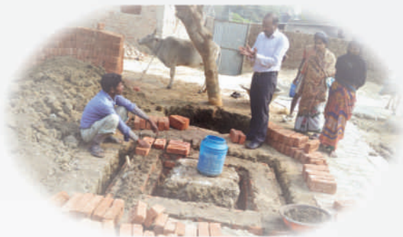
Individual toilet under construction in a slum
